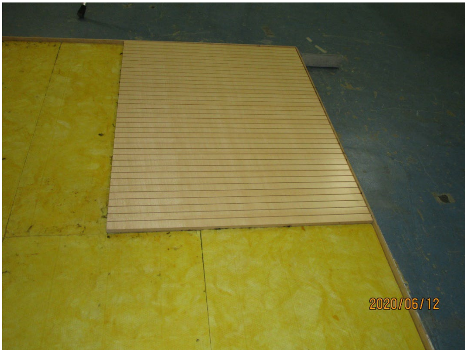
Figure 2 – Grooved panel layer partially installed, fiberglass base layer
